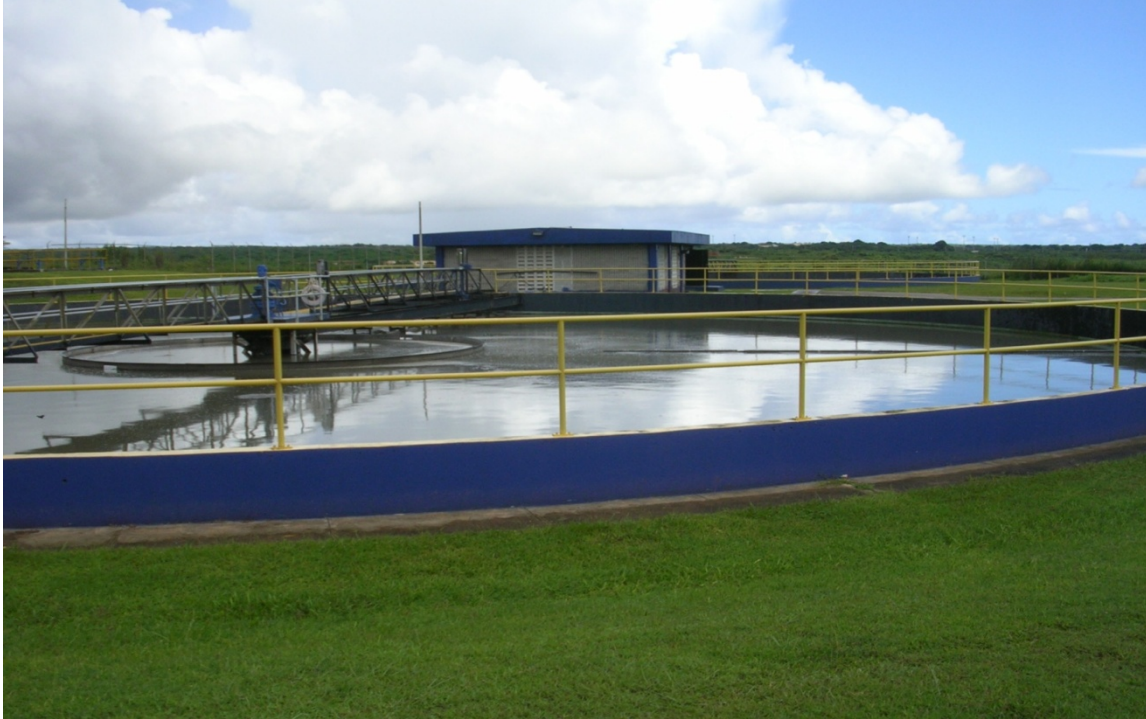
Figure 12. Northern District Wastewater Plant
