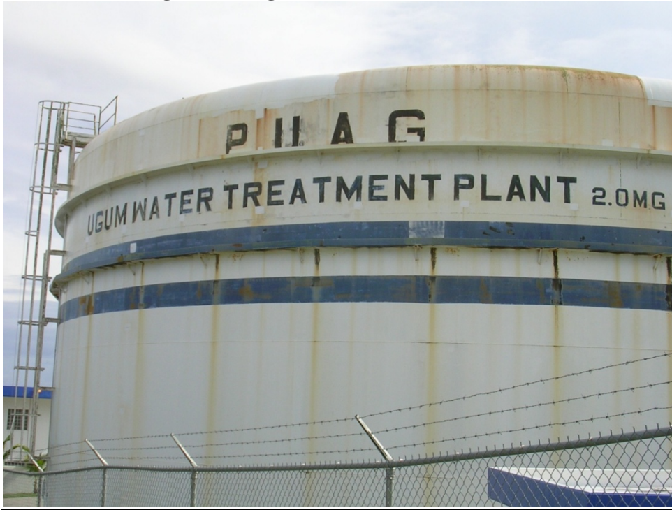
Figure 11. Ugum Water Treatment Plant
