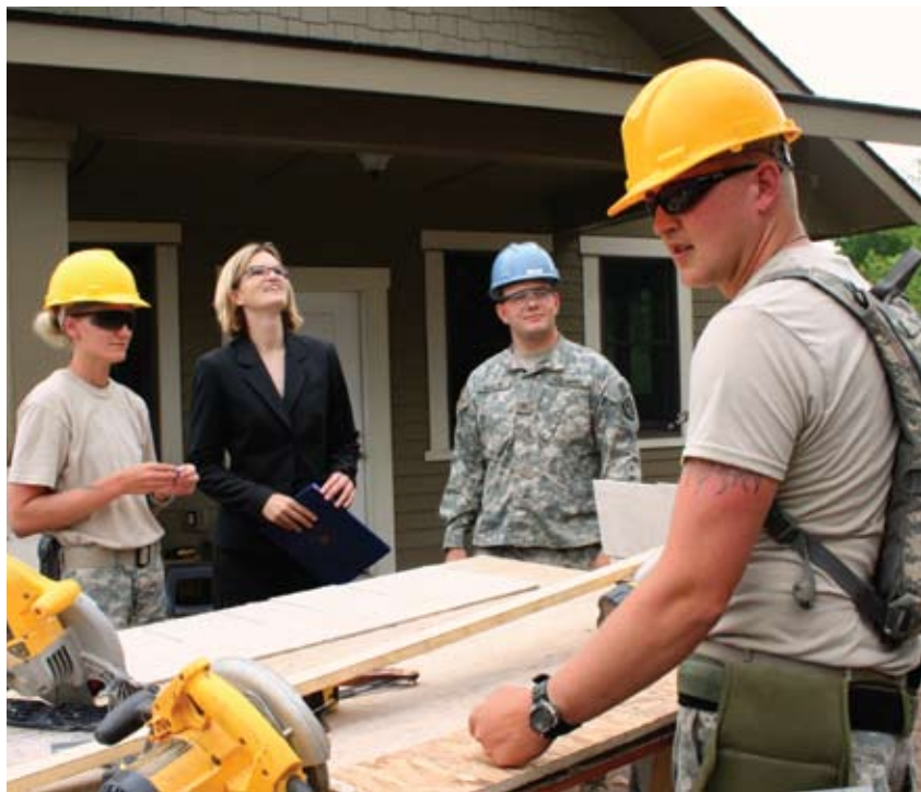
Members of the 851st Vertical Engineer Company and other visitors inspect new buildings at the Disabled Veterans Rest Camp, June 24, 2009.
