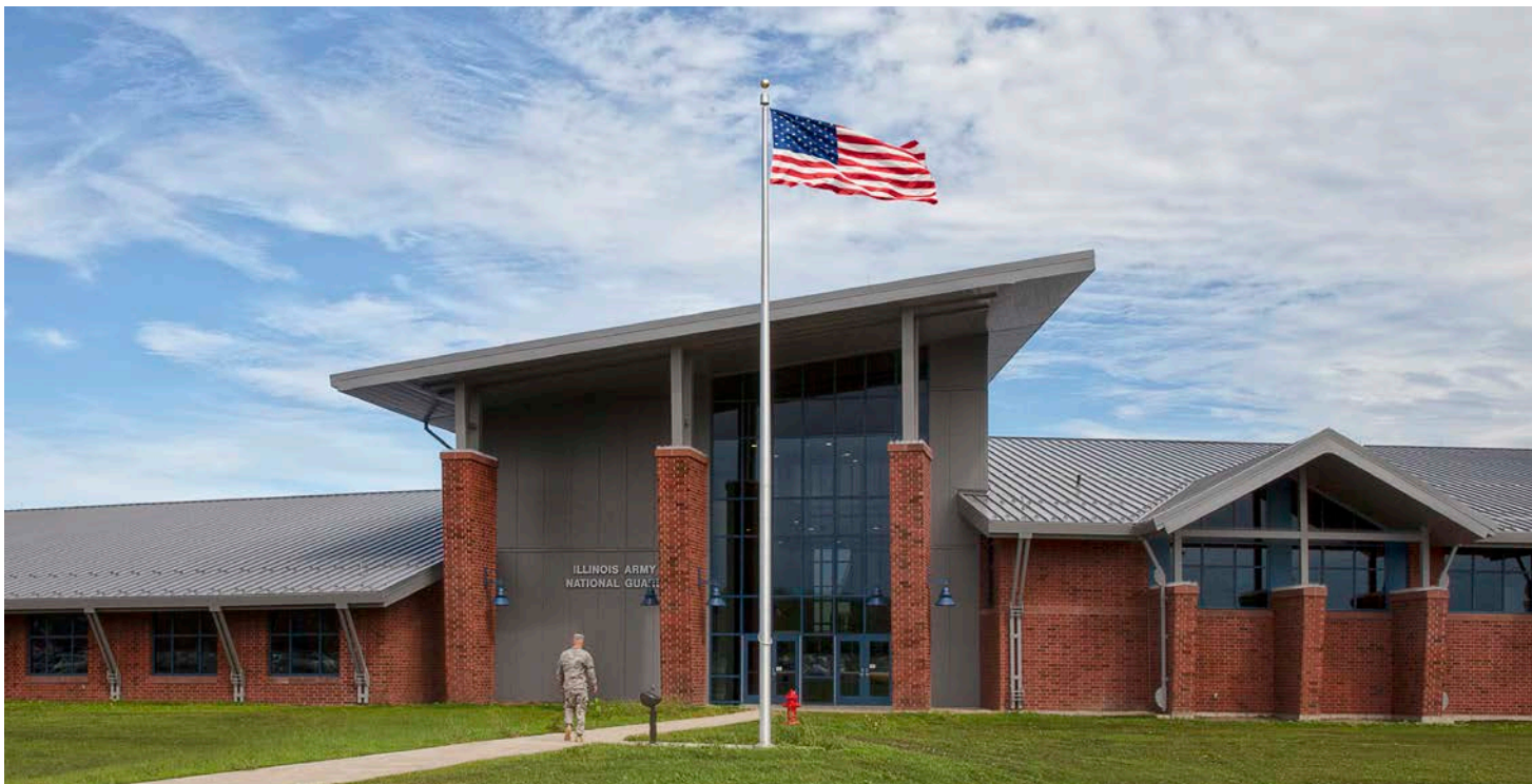
The Illinois Army National Guard Readiness Center was developed as a partnership with the Heartland Community College in Normal, Illinois. The readiness center was designed with a single story wing for public accessible entrance to the main level for access to the common authorized areas of classrooms, kitchen, and latrines. The opposite two-story wing supports the Illinois Army National Guard with a secured entrance to administrative space, staff sections for operations, secured equipment locker rooms, male and female latrines with showers, and a simulation room. (Photo courtesy of Illinois Army National Guard)
