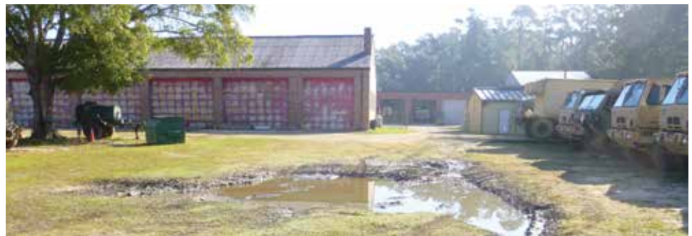
The photos above show the windows (top) and the motor pool, maintenance building, and parking (bottom) at the South Carolina ARNG’s Hemingway Readiness Center, which was built in 1956.
