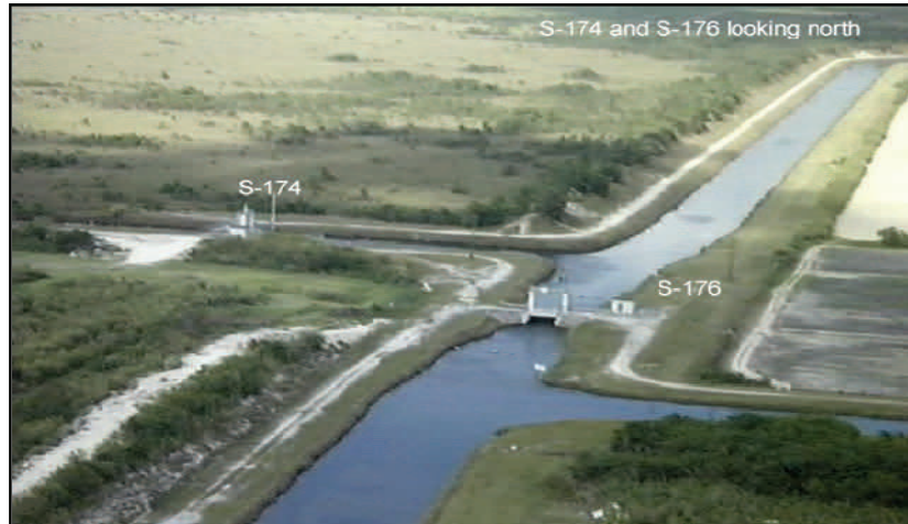
C-4 Canal System in south Florida
