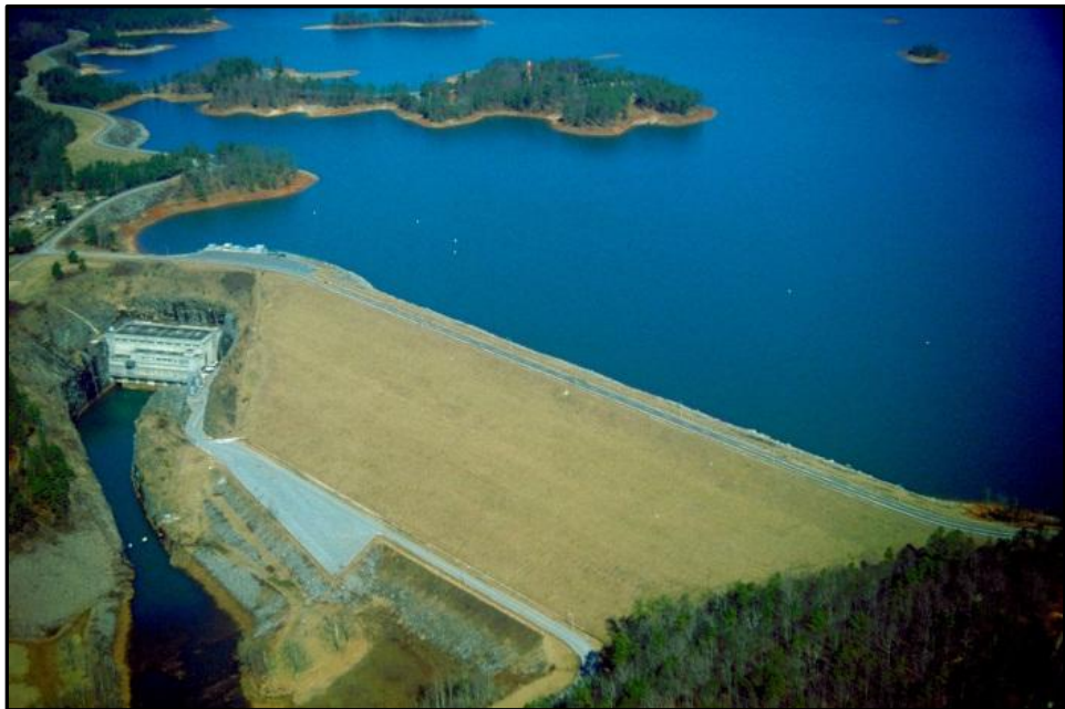
Figure 2. Buford Dam on the Chattahoochee River in Georgia (USACE)
