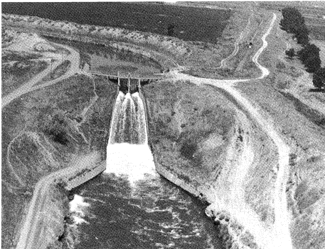
Figure 1-2. Vertical Drop on an Irrigation Canal
