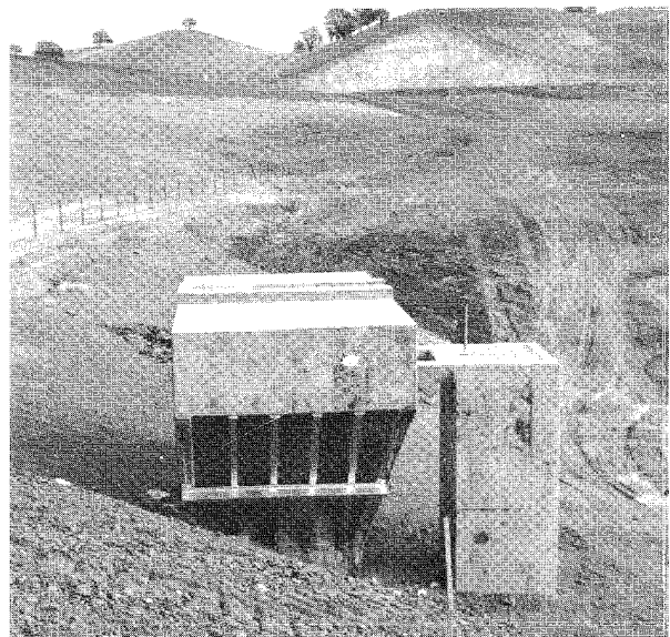
Figure 2-16. Intake structure of low-level outlet works
