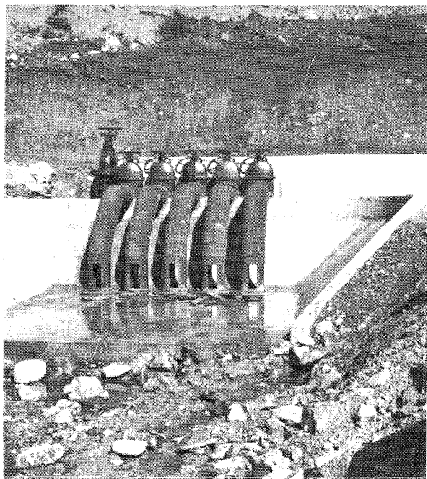
Figure 2-17. Terminal structure of outlet works
