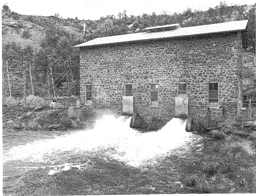
Figure 1-2. South Power Plant located on Bottle Creek, California with a capacity of 4,000 kW. Constructed in 1910. (Courtesy of Pacific Gas and Electric Company).
