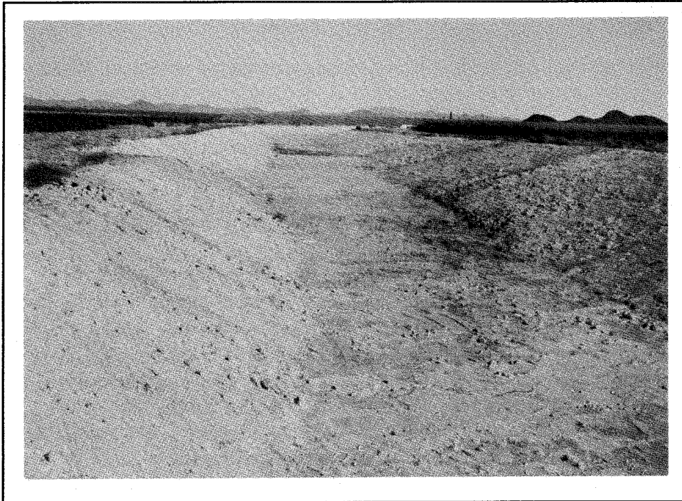
Figure 2-3 Lined Diversion Channel, Looking Upstream Toward FRS
