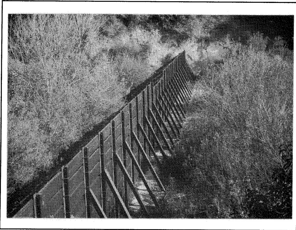
Figure 3-1 Debris Barrier Wall in Southern California
