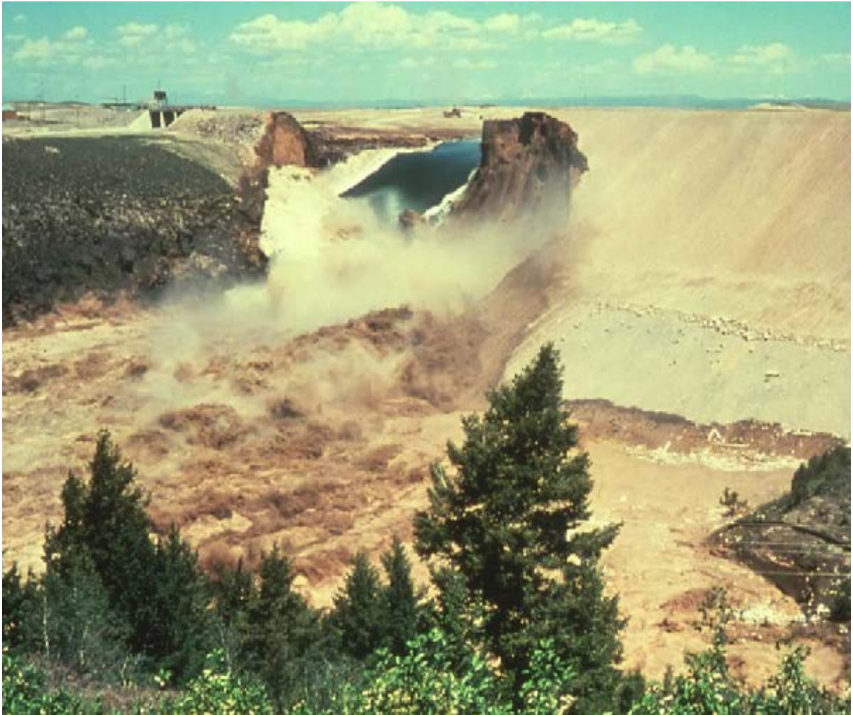
Figure 14-16. Significant Turbulence and Sediment load during the Teton Dam Failure
