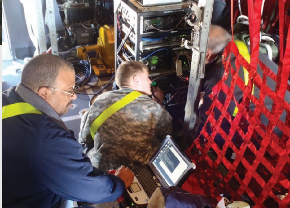
ARL engineers working with a Soldier while installing the system on an aircraft.
