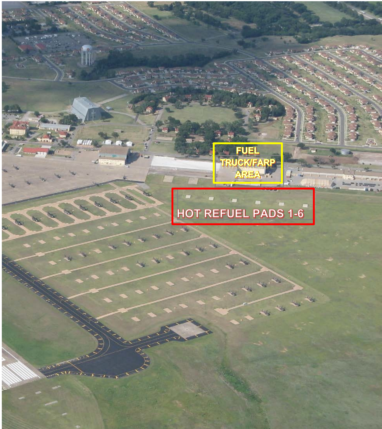
Figure 6-1. HPAAF Rapid Refuel Area (Tactical)
