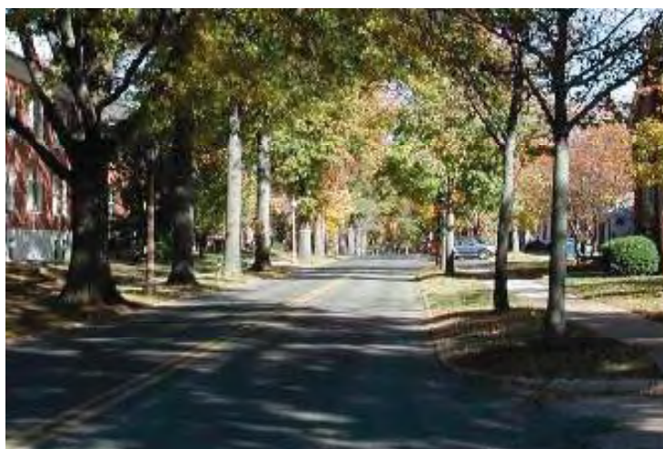
Example of a secondary road on Fort Belvoir (21st Street, Fort Belvoir)
