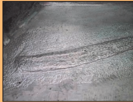
Localized crack repair treated with UIT.
