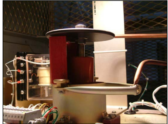
The Legacy ignitron crowbar device.
