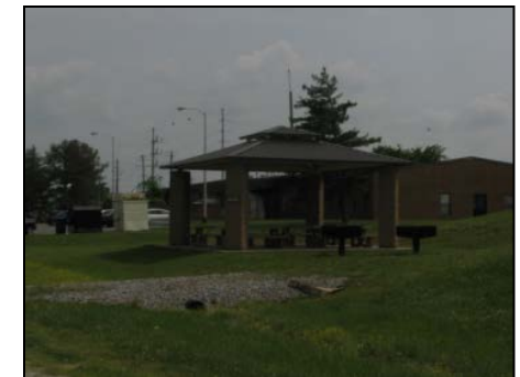
Industrial Use Shelter
