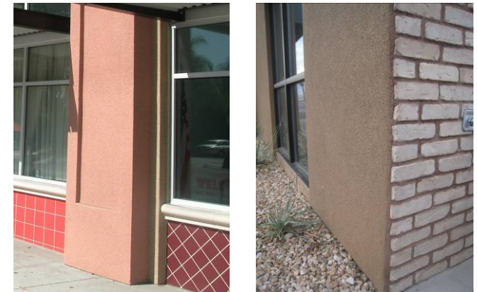
Figure 12. Materials that change on inside corners (above left image) and on outside corners (above right image)
