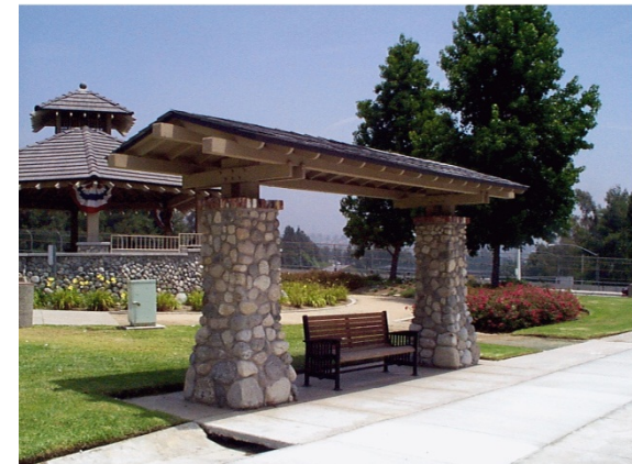
Bus shelter with bench
