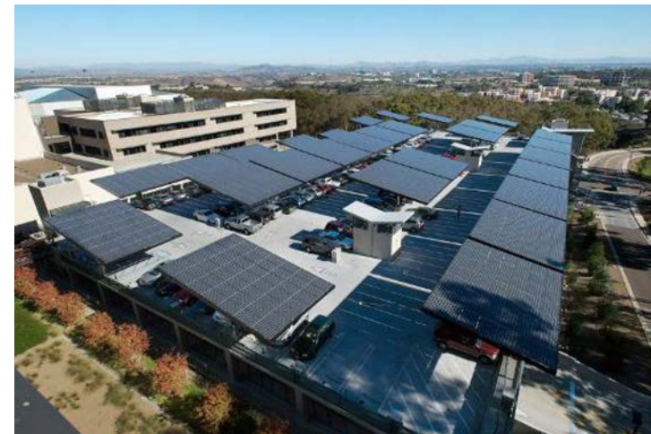
Solar panels on awning (above left image) and roof (above right image)
