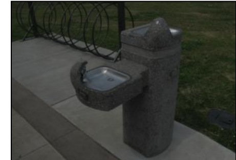
ADA accessible drinking fountain
