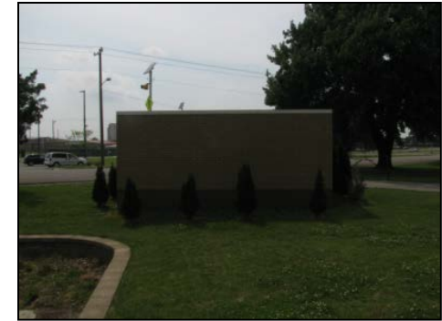
Dumpster screen wall with landscaping and retention wall
