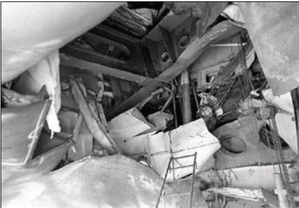
Estimated to cost about $1,500, an unsophisticated contact mine that was based on a 1908 Russian design caused some $96 million in damage in 1987 to the frigate USS Samuel B. Roberts, shown above with damage to the hull as seen from dry dock, almost causing the ship to sink.
