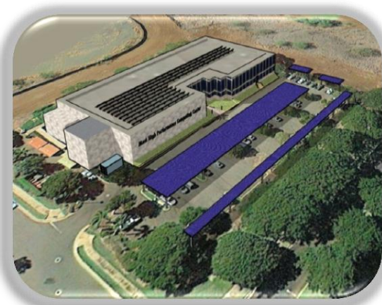
Maui Advanced Energy Storage #1, 3, & 4
