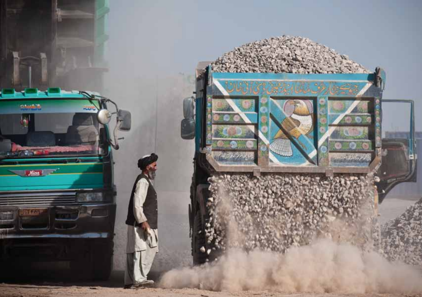
A local-national truck dumps gravel in Afghanistan. Local national contracts awarded by the regional contracting command were one source of labor for construction projects.
