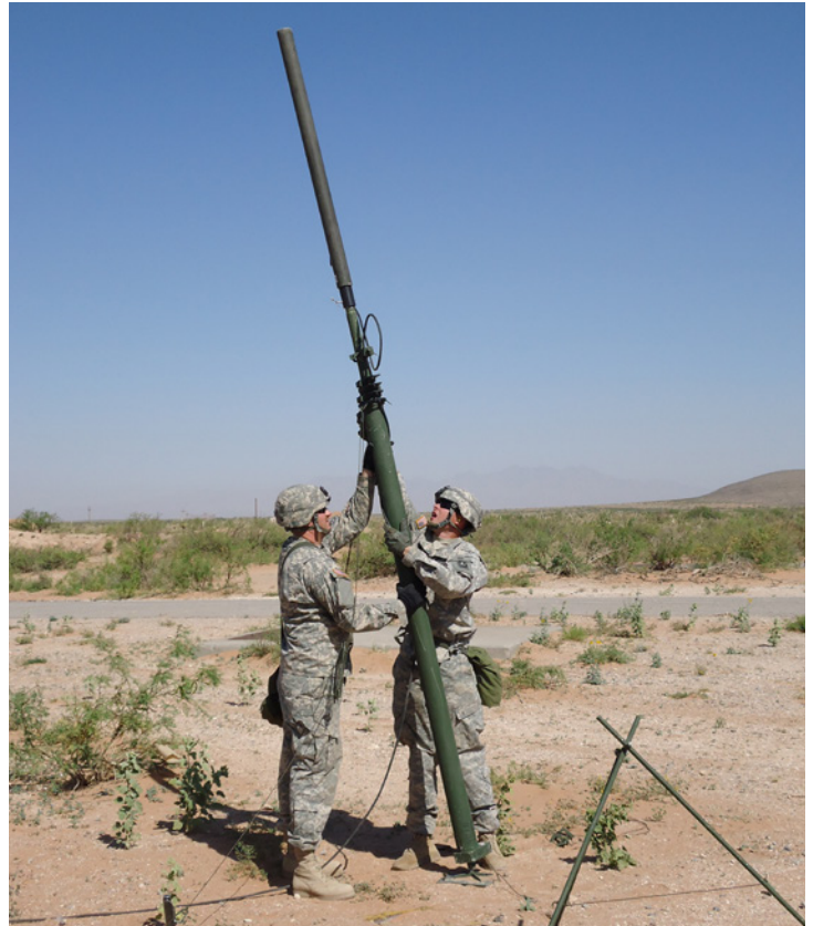
Soldiers from A Battery, 4th Air Defense Artillery, deploy an antenna mast. (Photo courtesy of A BTRY, 4th ADA)
