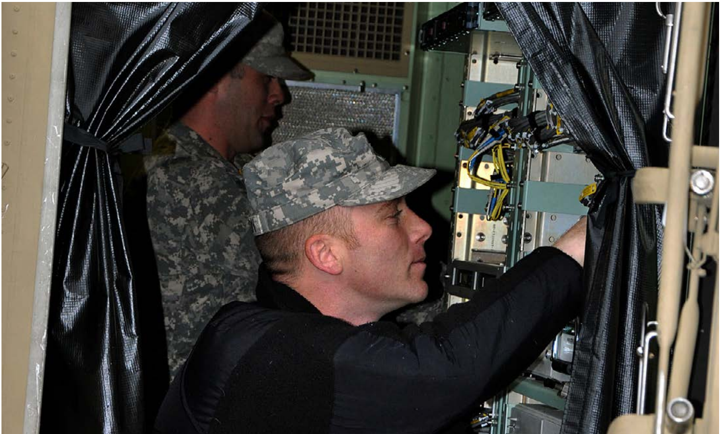
SGT Michael Norton and CPL Eric Cook, with the 41st Fires Brigade, setup communication equipment connected to the joint network node during the unit's communication exercise at Fort Hood, Texas. The Soldiers provided support for the 41st Fires Brigade and the 17th Fires Brigade based out of Fort Lewis, Wash. (Photo by SGT Kyle J. Richardson, U.S. Army)
