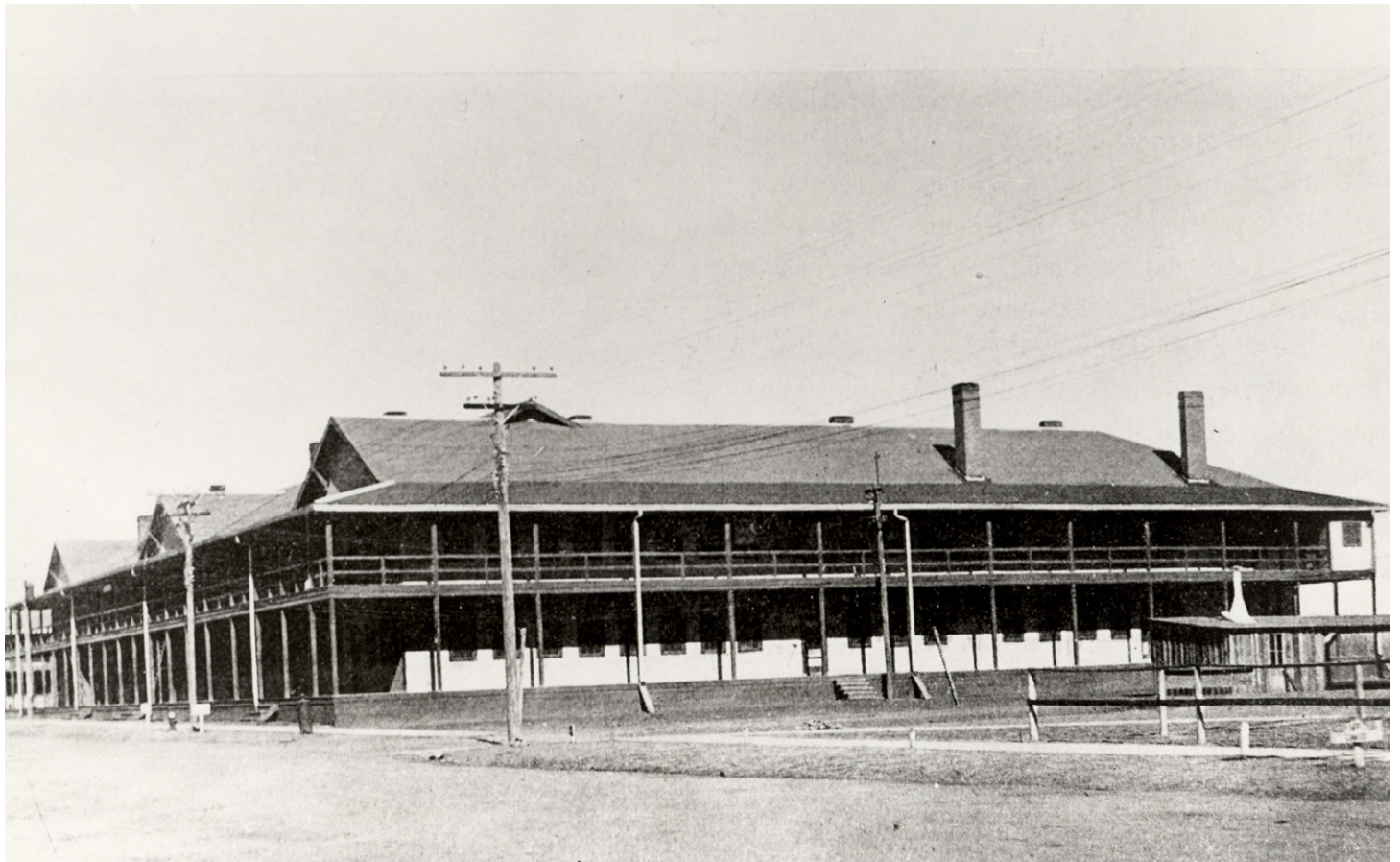
Old Snow Hall, the ‘Hub of the American Artillery Wheel,’ in 1922. It was a large two story wood framed building with porches on both floors. This photograph was taken shortly before the building burned. (Photo Courtesy of the Fort Sill National Landmark Museum)
