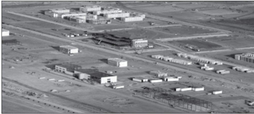
The brigade combat team (BCT) construction development on Fort Bliss, Texas, will include infrastructure and facilities for six BCTs. (Photo courtesy of Office, Chief of Air Defense Artillery, Fort Bliss)
