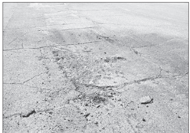
A 122-mm rocket was fired at high angle and detonated on a street in Baghdad, as shown here, on 6 March 2005.
