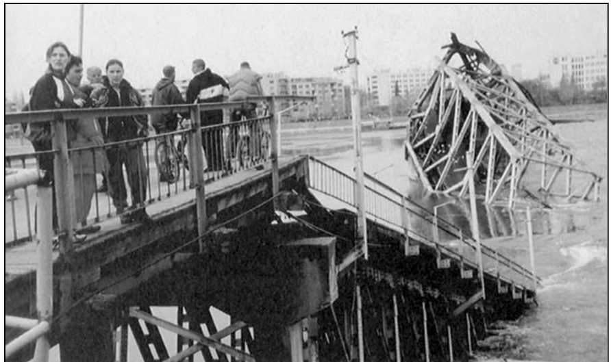
The question for the targeting team and the commander is whether or not the value of the target outweighs the collateral damage that might be caused by the deaths or injuries of civilians fleeing across a bridge, such as this bombed bridge in Kosovo.
