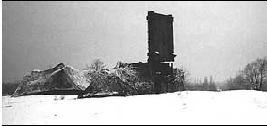
The 10th TAD's Q-37 radar "watches" quietly in the snow at Fort Drum for enemy fire.
