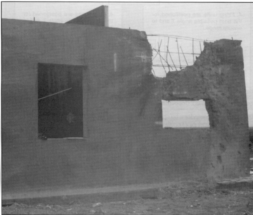
This picture shows the effects a Copperhead round has on a reinforced concrete building.
