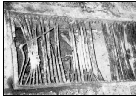
Top: East German soldiers' washroom. Middle: Rotten pipe insulation. Bottom: Broken pieces in the cellar floor where rats come in.
