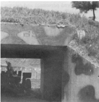
This ROKA 105-mm howitzer in a concrete bunker is aimed at the DMZ. Notice the thickness of the overhead cover.
