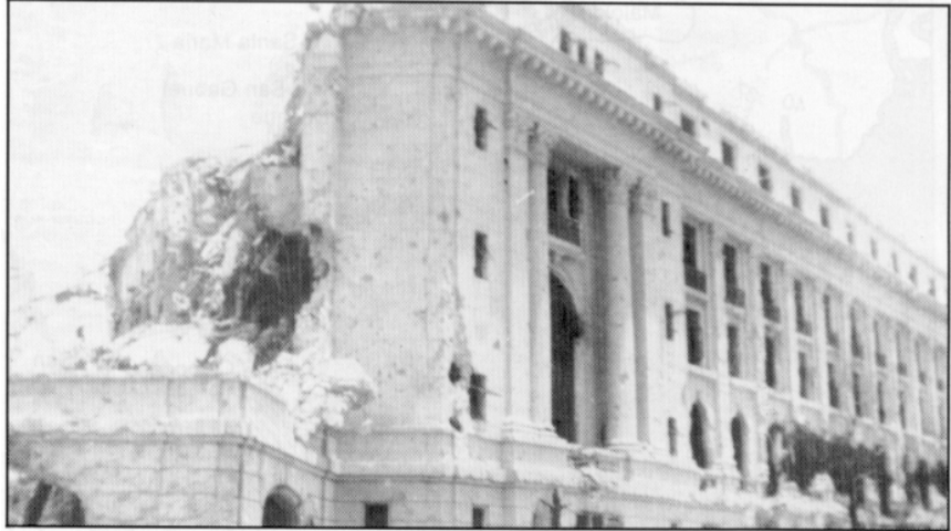
Large governmental buildings in Manila showed the effects of prolonged artillery fire.
