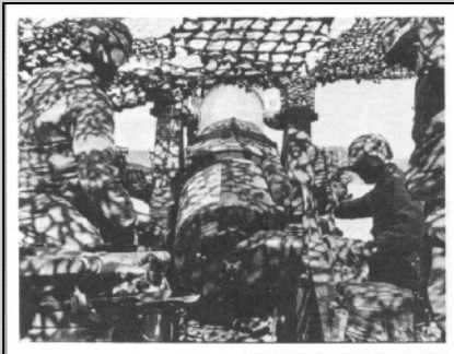
Bubbles Level—8-inch steel is on the way.
