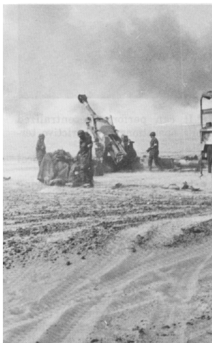
The inclusion of M198 towed 155-mm howitzers gives maneuver commanders more fire support assets.
