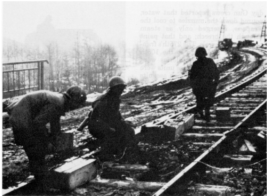
Engineers prepare a railroad bridge for demolition.
