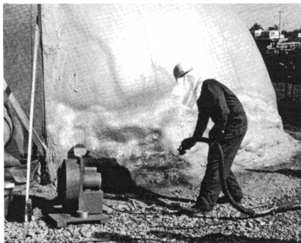
A CERL engineer sprays foam onto the shell.
