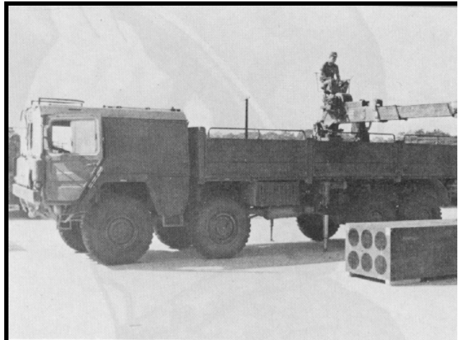
A German MAN vehicle loads a general support rocket system (GSRS) launch pod/container simulator during evaluation at the Army Missile Research and Development Command. The German truck, along with vehicles from Lockheed and Pacific Car and Foundry, is being assessed for the GSRS ammunition resupply mission. MIRAD-COM is also studying the impact of GSRS on the ammunition supply system.
