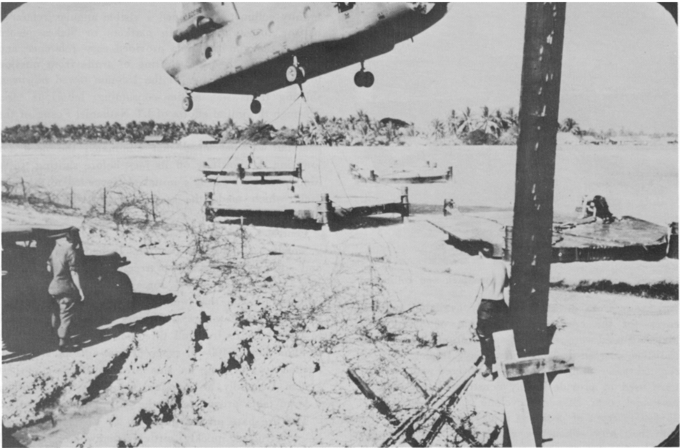
CH47 emplacing an airmobile firing platform. (Photo courtesy CPT N. King)
