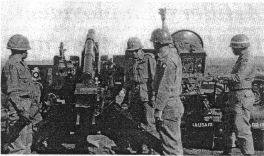
Figure 1. M36 chronograph emplaced to measure muzzle velocity of a 105-mm howitzer.
