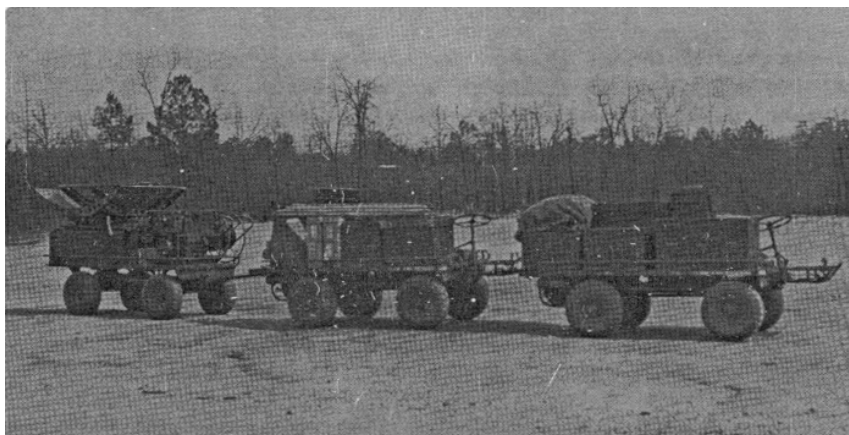
Figure 6. Reduced metro section prepared for airlift.
