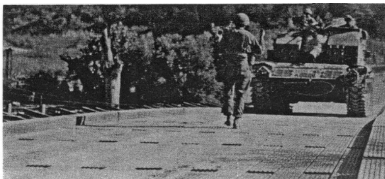
Figure 5. Self-propelled howitzer using M4T6 bridge.
