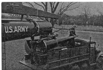
Figure 19. The warhead section is hoisted from its container and attached to the rocket motor with four bolts. Left.
