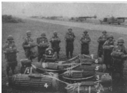
75mm howitzer section ready for loading, Note control lines tying complete load together.
