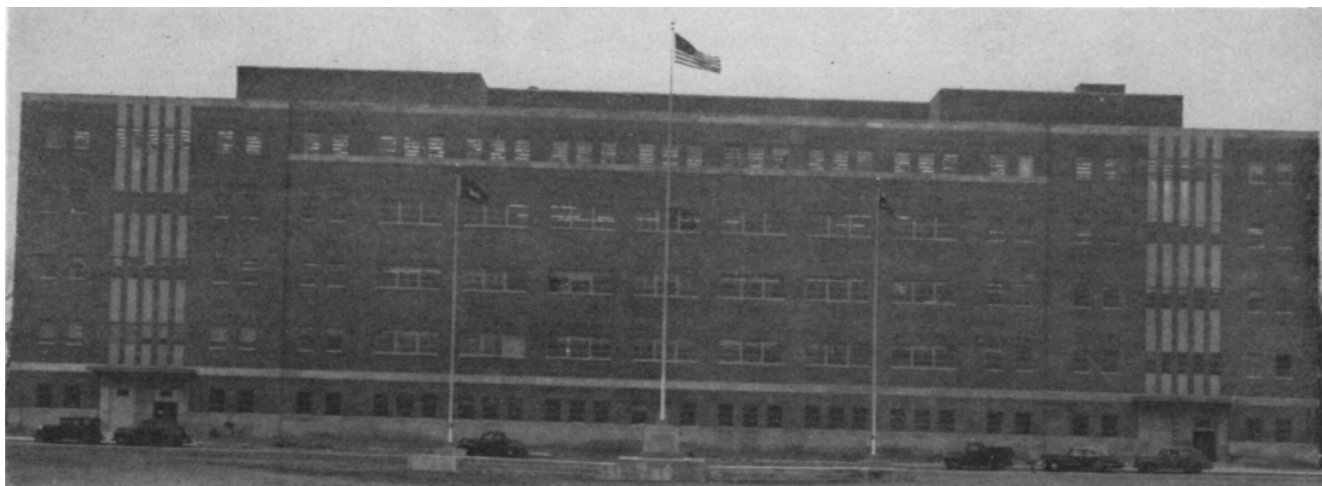
The home of the Army Map Service on MacArthur Boulevard in Washington, D. C.
