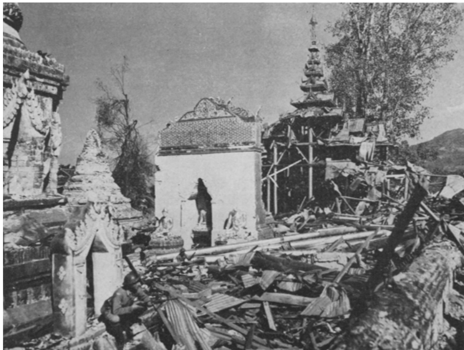
Counterbattery against Namhkam resulted in the almost complete destruction of this large Burmese temple in the center of the city.
