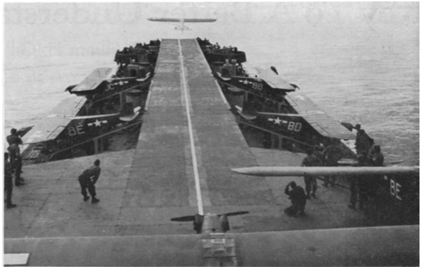
Ten cubs can be carried aboard an LST: six along the runway and four in cradles. The runway, 220 feet long and 16 wide, is used for take-offs only.
