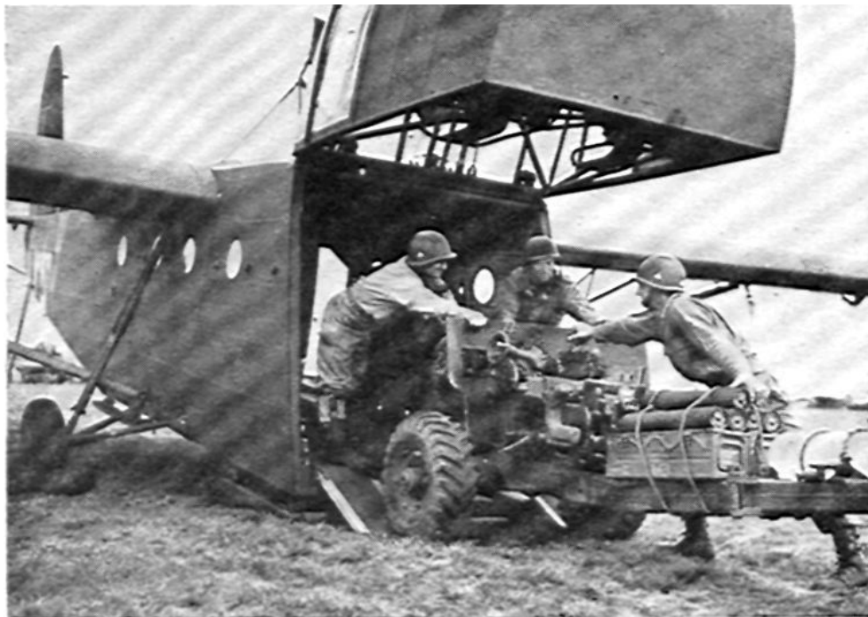
Three members of the Allied airborne army that took part in the assault on Holland load a 57-mm gun into a glider. Notice how much space is saved by lashing ammunition and equipment onto the trails.
