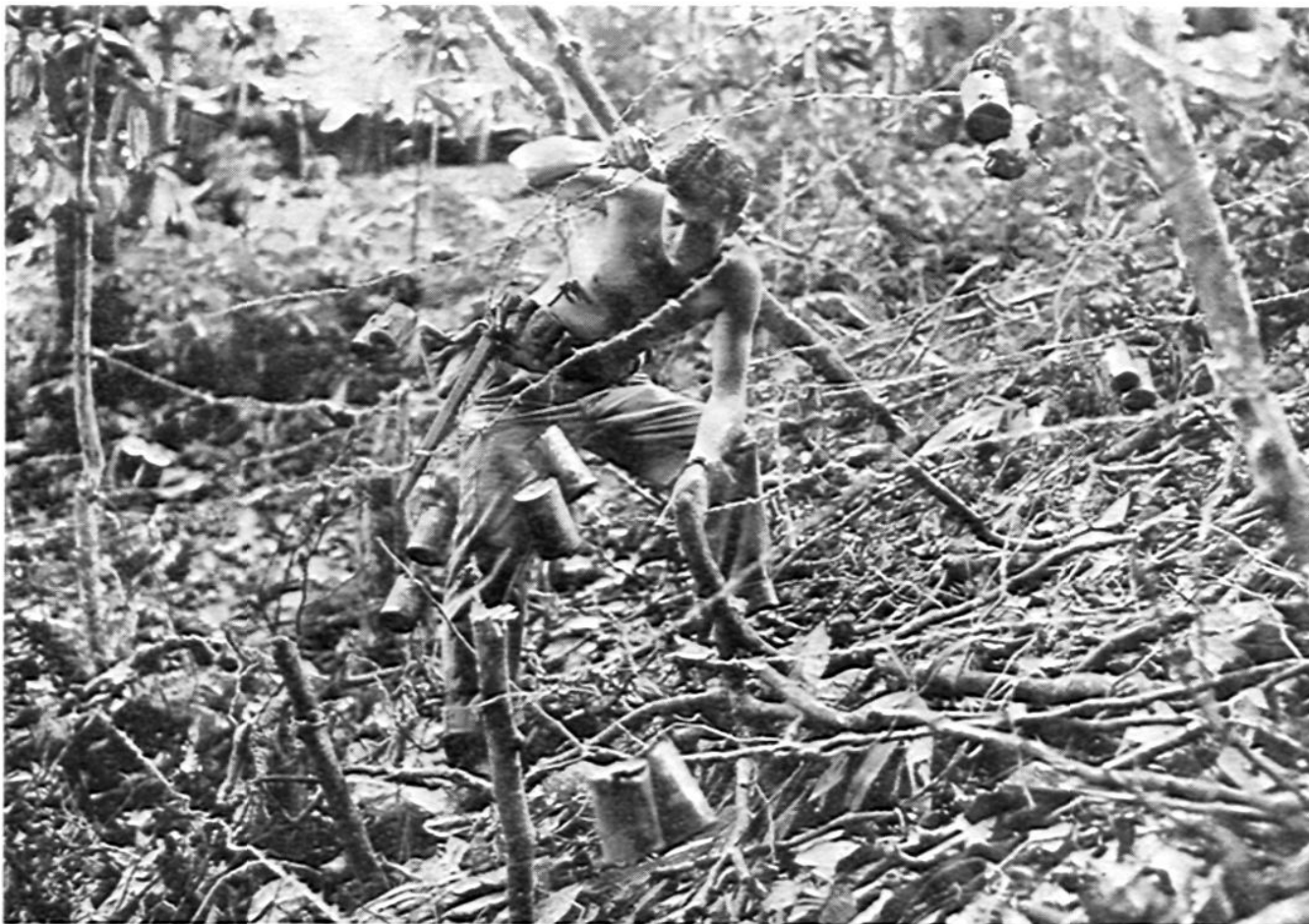
A double apron barbed wire fence, well hung with warning cans, along the perimeter of Company E, 145th Infantry, 37th Division, on Bougainville, in March, 1944. Next day the Nips began the
