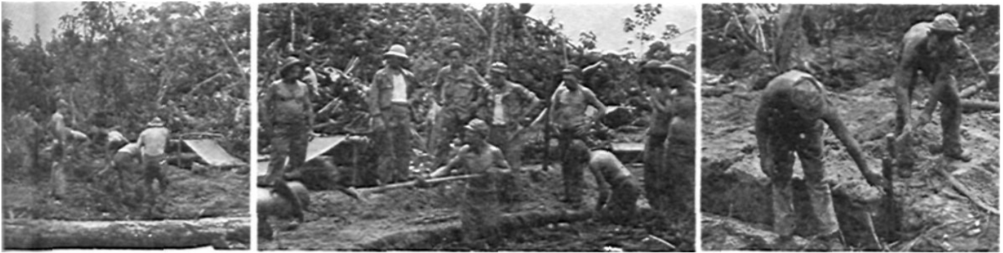
Trail trenches and logs were essential in this rainy area.
