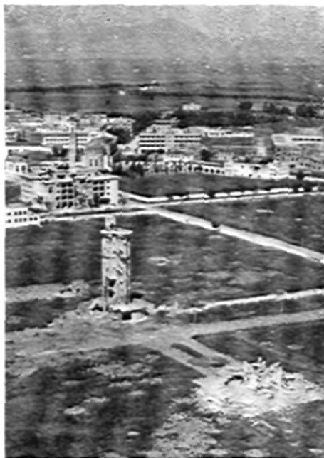
Tower 2 is standing. Tower 1 is a pile of rubble.
