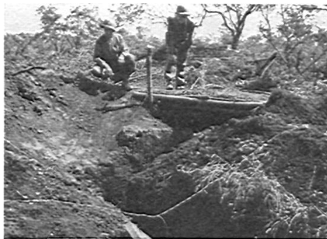
Dig 'em deep! The Germans do—we taught them that life is healthier that way. Trench shown here leads into a German 152-mm gun emplacement. A system of deep trenches and dugouts ran throughout the area of this 3-gun battery position.
