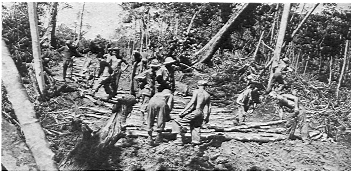
In the pursuit to Zieta, later in the campaign, jungle mud compelled extensive corduroying of the newly hacked roadway.
