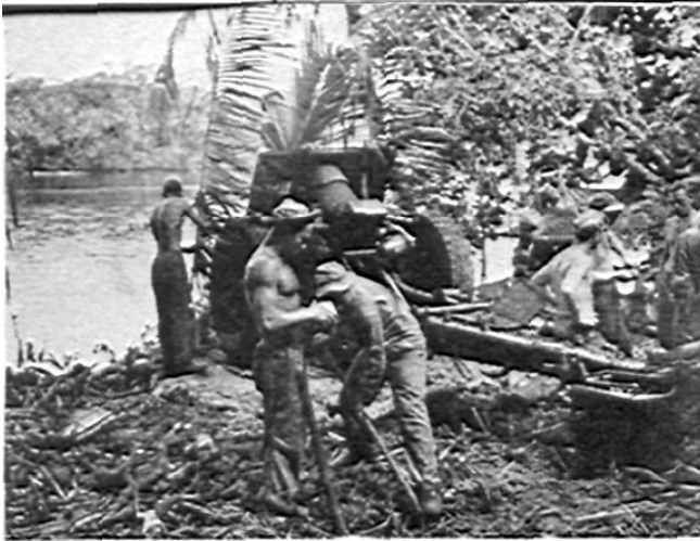
Positions are organized quickly. Trail trench is dug promptly, and camouflage immediately placed in front of exposed pieces.
