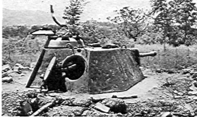
In the Libyan desert the Germans strengthened their defensive positions by digging in damaged tanks so as to constitute armored dugouts, with only the turret above ground. In Italy they extended this method, embedding the turrets alone in concrete. Here is a PzKw-V turret with its 75-mm gun, near Pontecorvo; the flat area before it was liberally sown with all types of mines. Similar types of defenses can readily be installed in cities.
