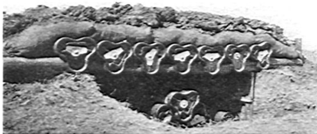
Figure 1. Ammunition shelter using dirt-filled fiber containers to support sandbag cover.
