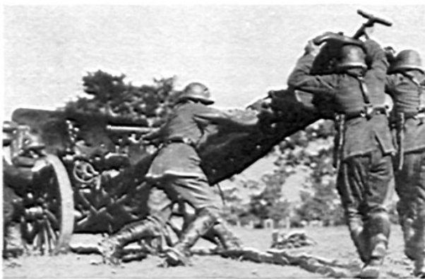
Emplacing the howitzer: modified box trail is well elevated for swinging, and then for embedding the hinged spade as much as possible.
