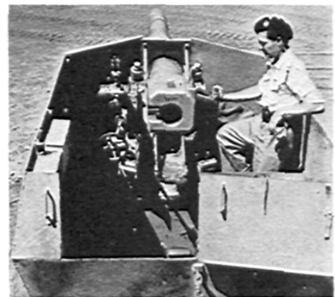
Reloading preliminaries: man at right has the charge in its short brass case, the next one carries a 1914 pattern short shell.
